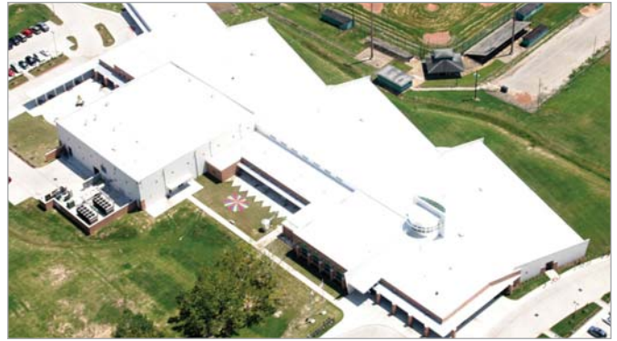
Flex Elvaloy ® KEE Roof Systems are very popular with Schools, Colleges and Universities.
