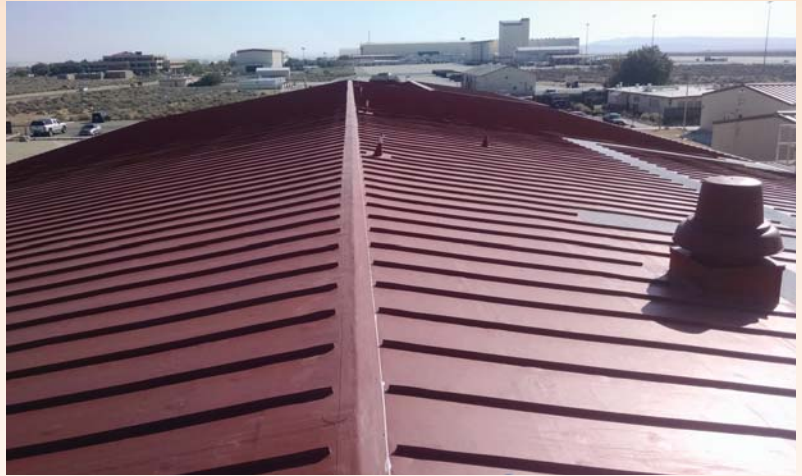
The product's base flange is approximately 2" wide and the rib profile is 1-1/8" high. Each rib has an 1/8" diameter fiberglass reinforcing cord built in for dimensional stability.
