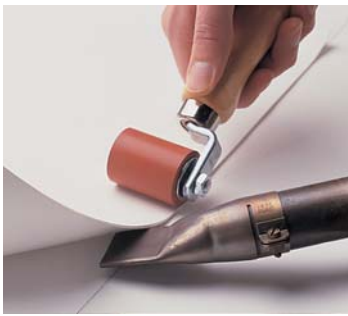
Flex roof membrane seams are hot-air welded. No solvents, glues or tapes are required.
