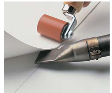
Flex membrane seams are sealed with hot-air guns, or special solvent.
