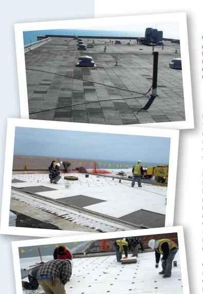
With RhinoBond, all fasteners are installed in one operation. killing two birds with one stone. No separate insulation and membrane fasteners are needed.
