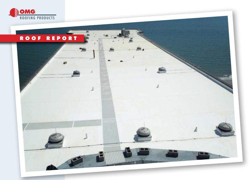
Tecta America Carolinas used the RhinoBond system to install a Flex Membrane MFR PVC roof on this 22-story condominium.
